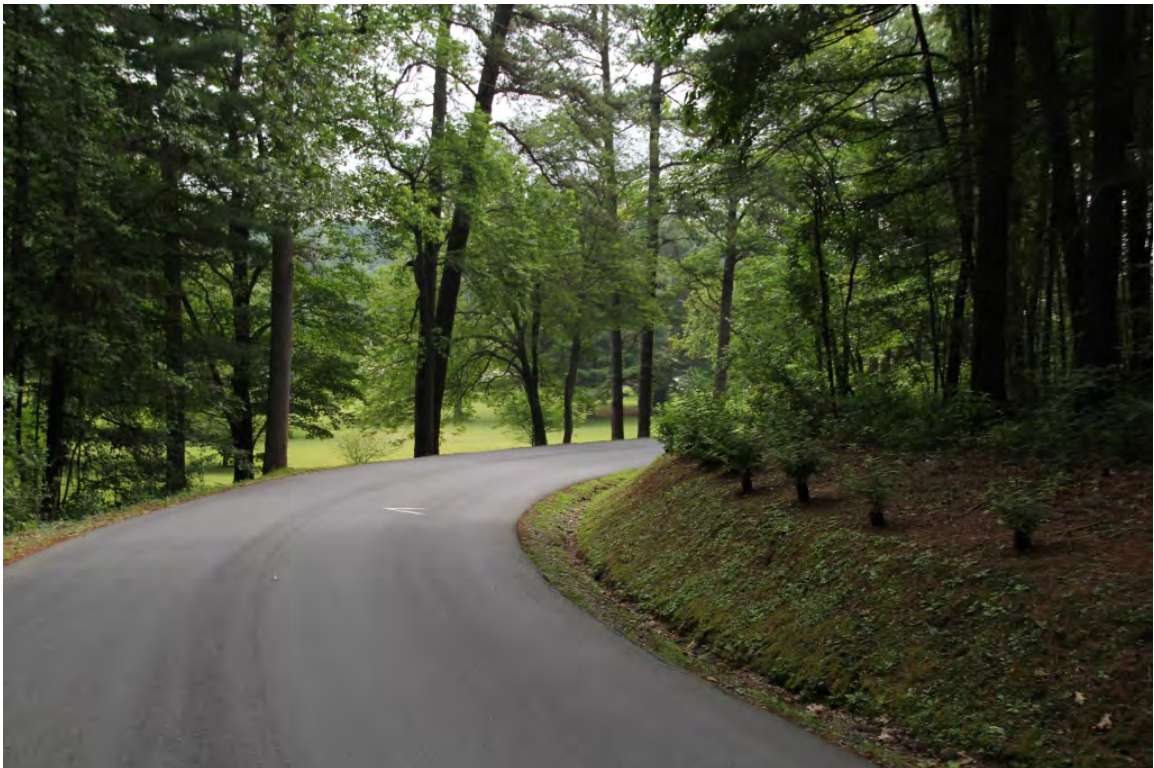
Lower Laurel Road, entrance drive, view to northeast
