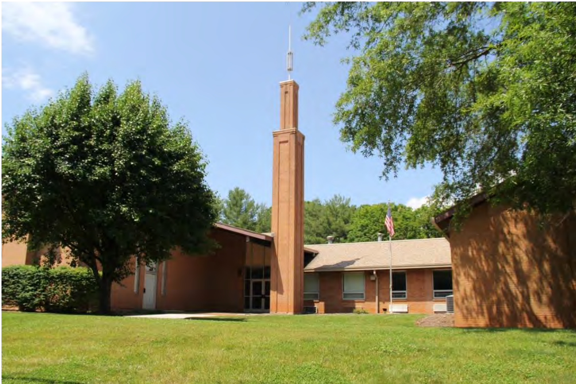
The Church of Jesus Christ of Latter-Day Saints Arden, 3401 Sweeten Creek Road, front view to southwest
