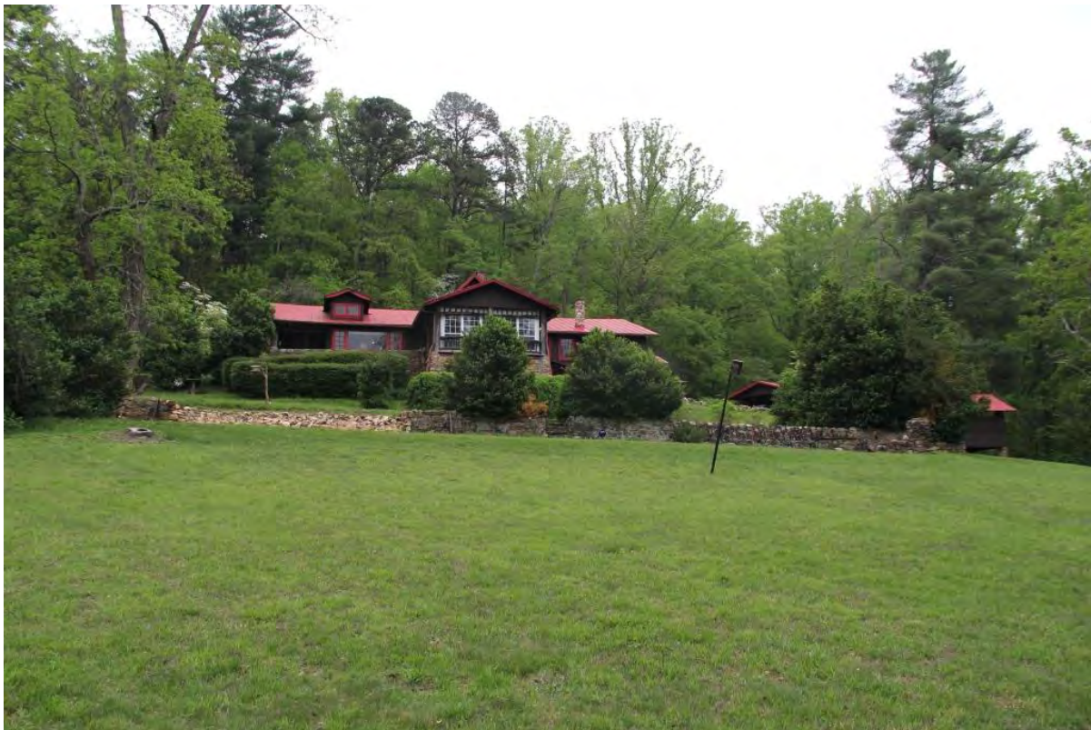
Round Top (Phillips Estate), 1663 Sweeten Creek Road, overall view to southeast
