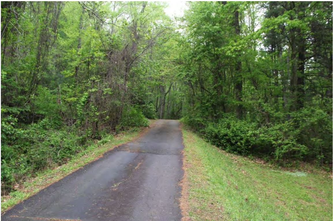
Carriage road, view to northwest
