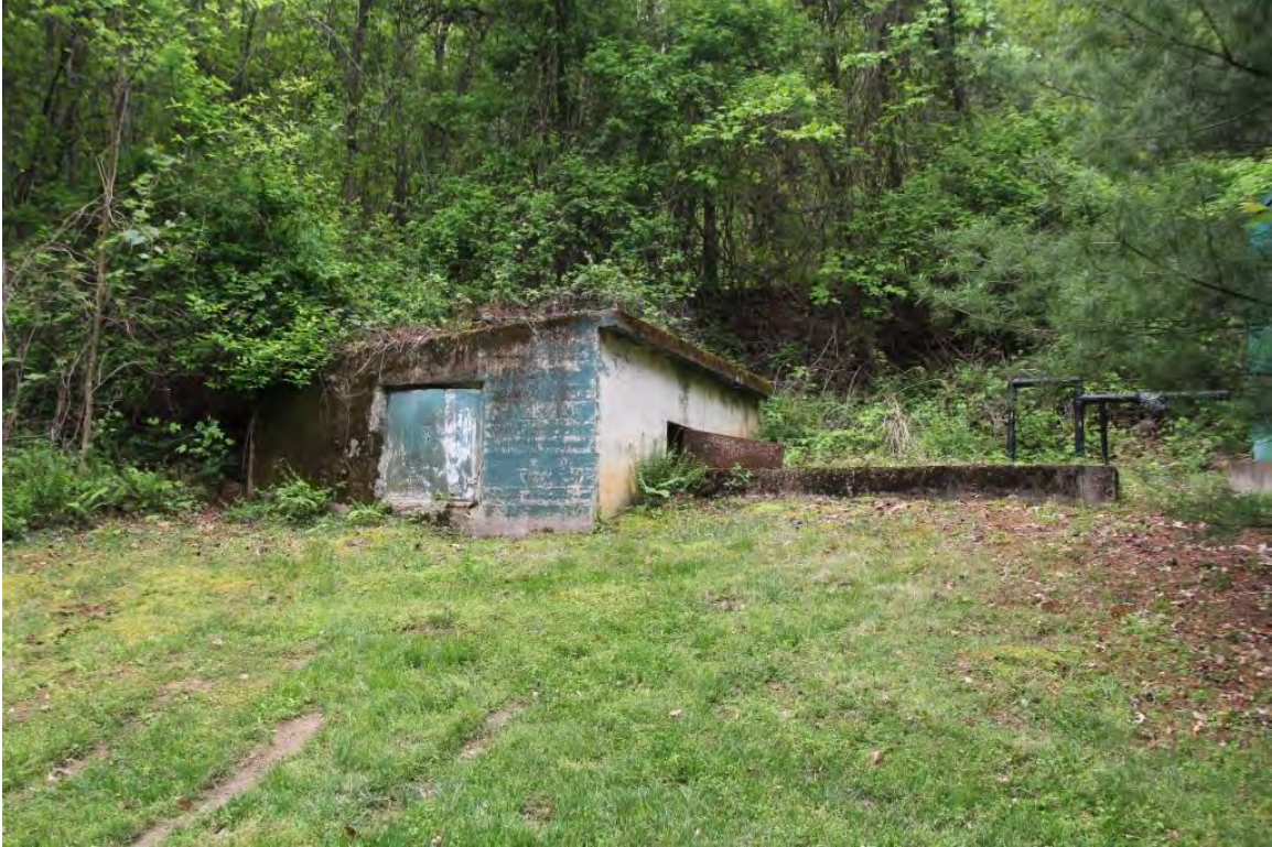
Reservoir (ruins), view to southwest
