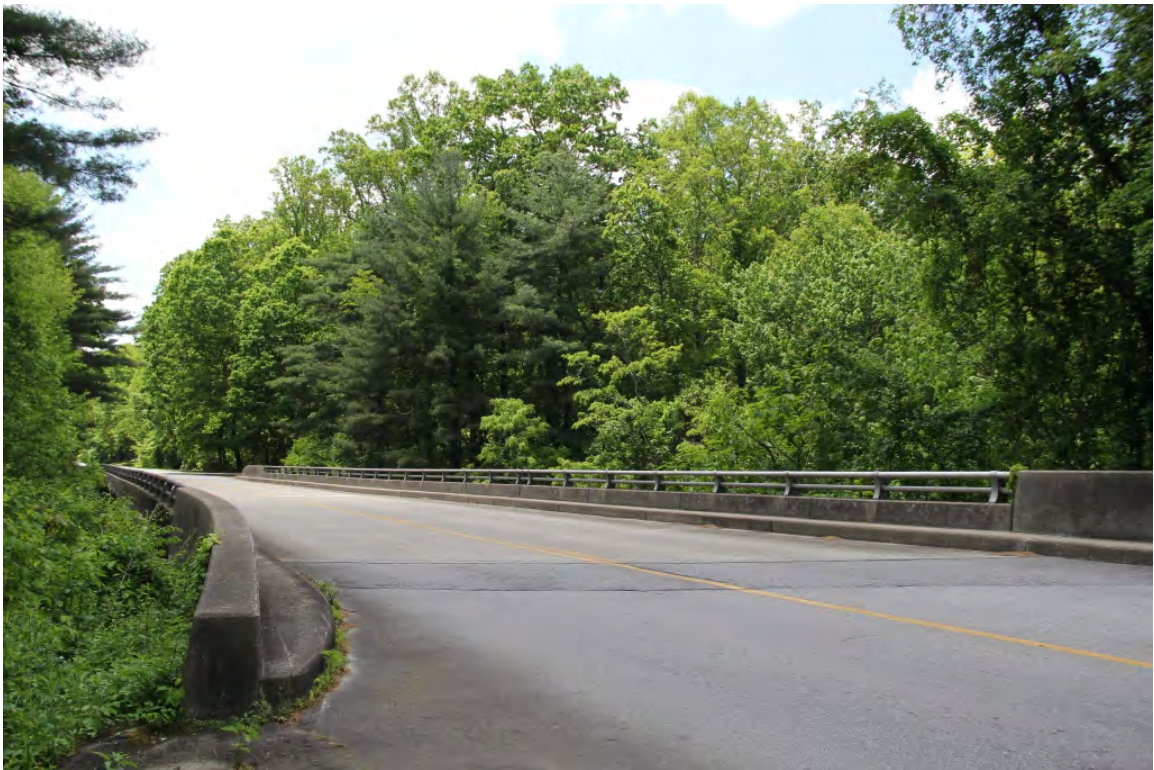
Blue Ridge Parkway, bridge over Sweeten Creek Road, view to east
