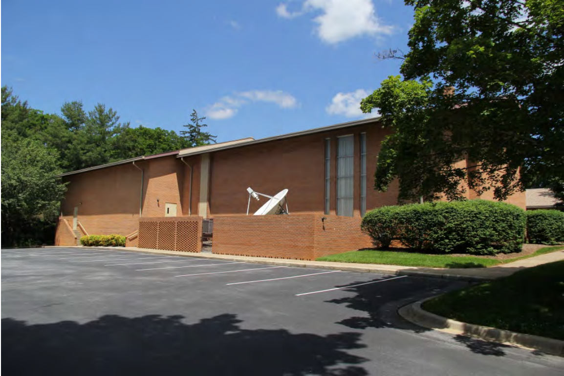
Arden LDS Church, chapel and gymnasium wing (1980s), view to northwest
