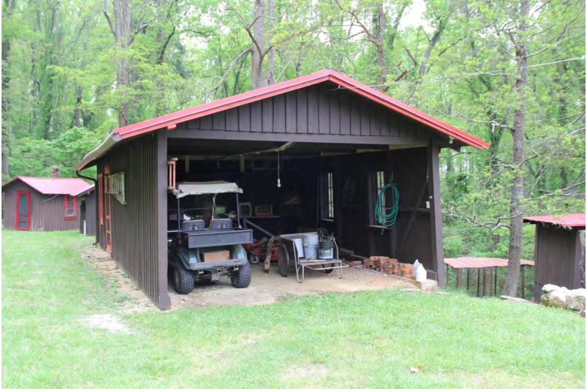
Garage, front elevation, view to south
