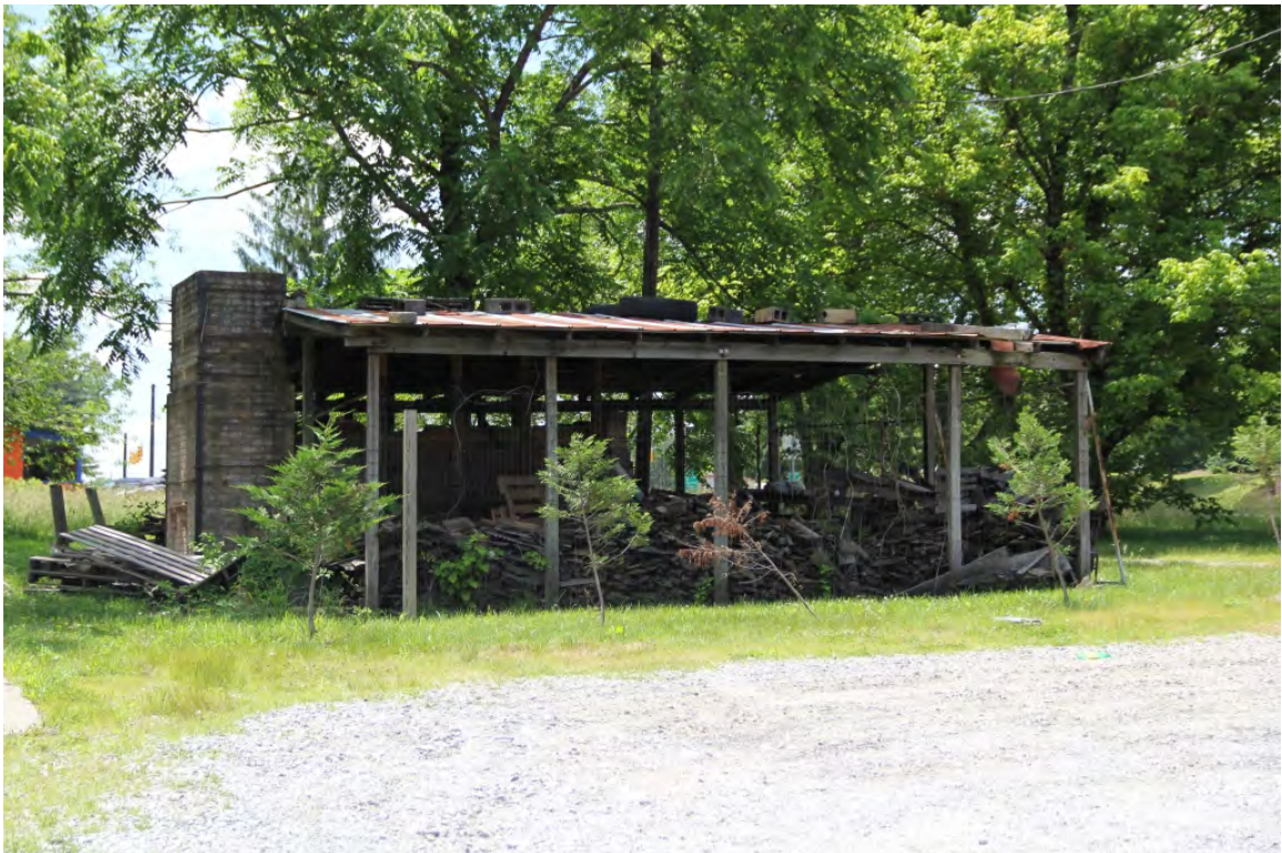
Kiln shed, view to south
