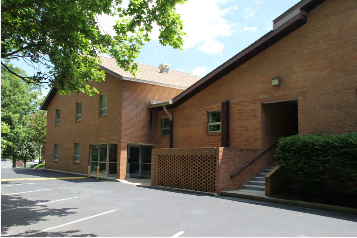
Arden LDS Church, gymnasium wing (r) and Family History Center (l), oblique rear view to northeast
