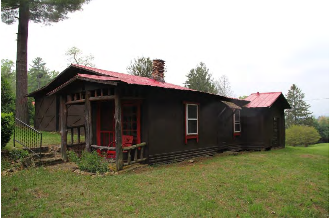
Garage, chauffeur's quarters, oblique view to southwest
