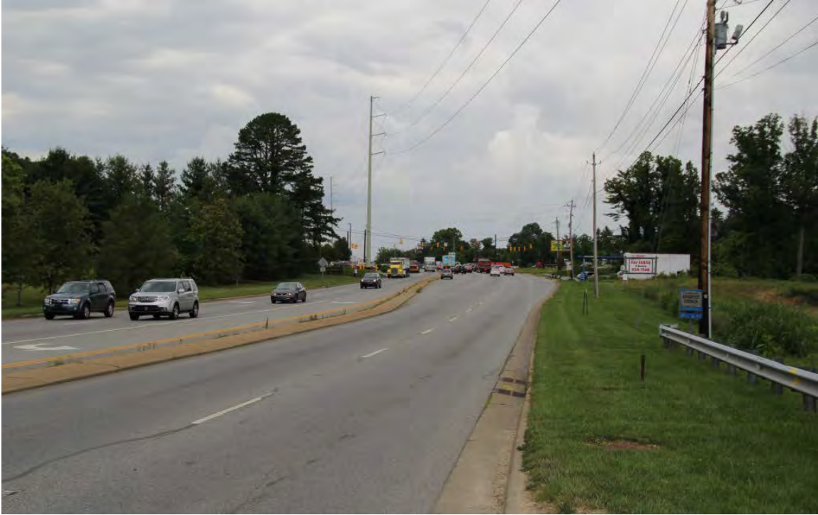
Hendersonville Road (US 25) near project beginning, view north to intersection with Sweeten Creek Road (US 25A) and Airport Road (NC 280)
