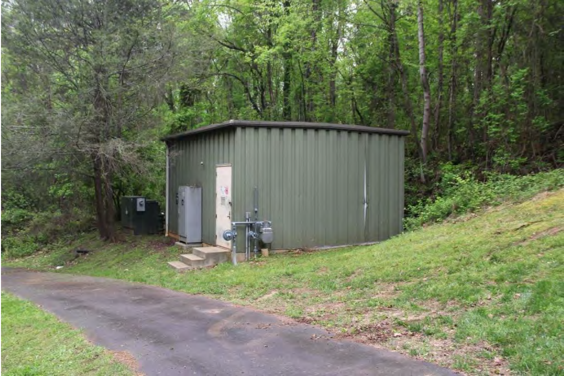
Maintenance Building (City of Asheville), view to southeast
