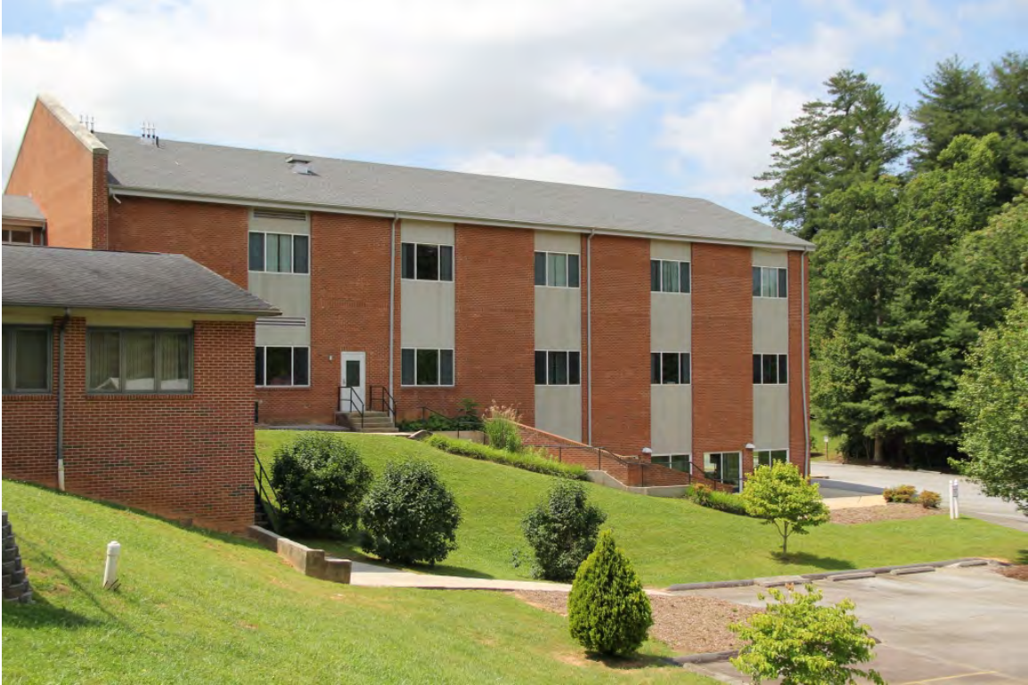
Youth building, north elevation, view to southwest
