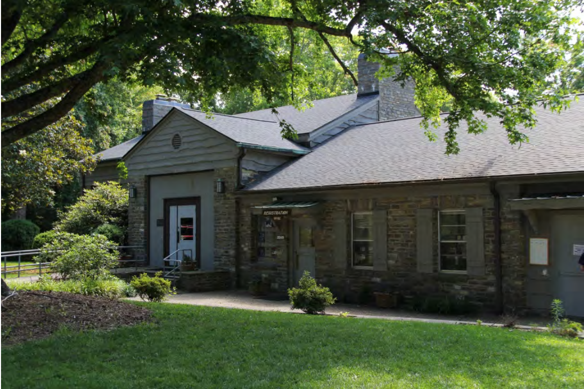
(#1) Efir Hall (1951), oblique view to east
