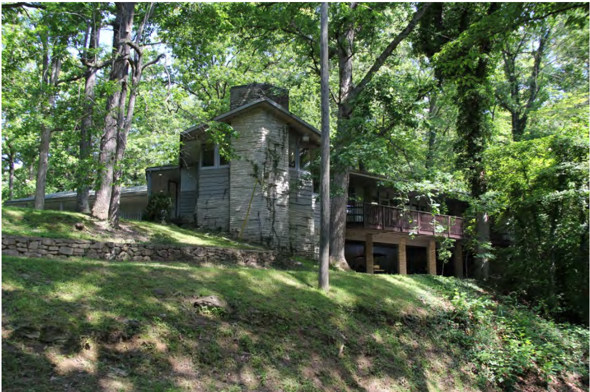
(#6) Mission Hall (1956), view to northwest
