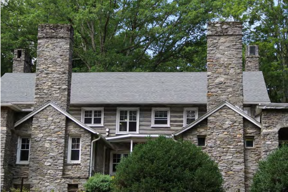
Givens House, rear elevation, view to southwest
