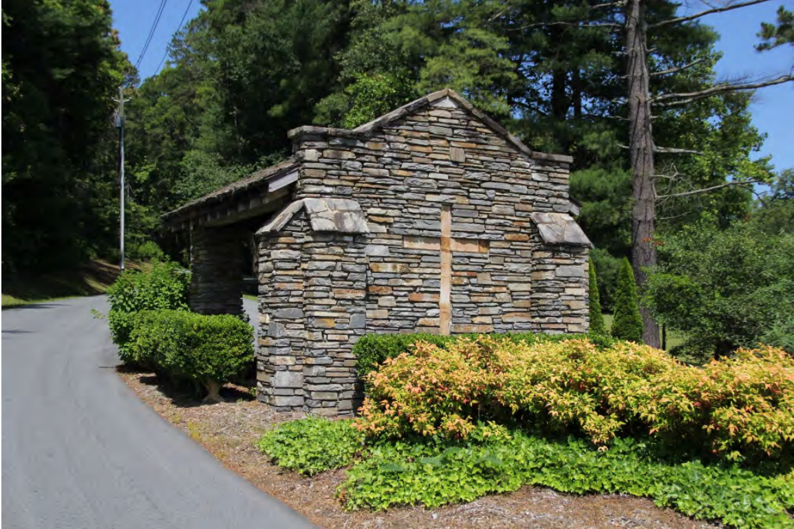
(#18) Gate House (1954), oblique view to northwest
