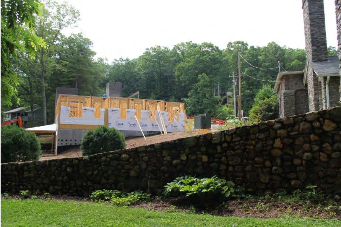
New construction southeast of Givens House, view to southeast
