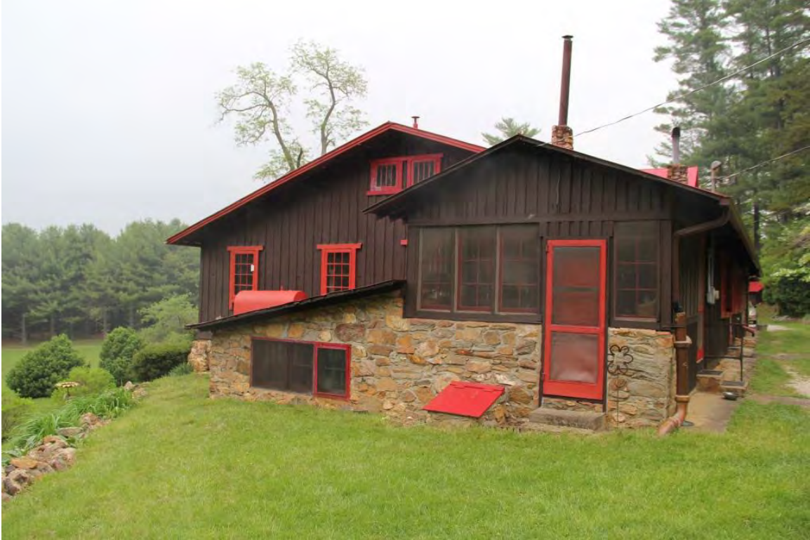
Horace W. and Emma Phillips House, rear elevation, view to north
