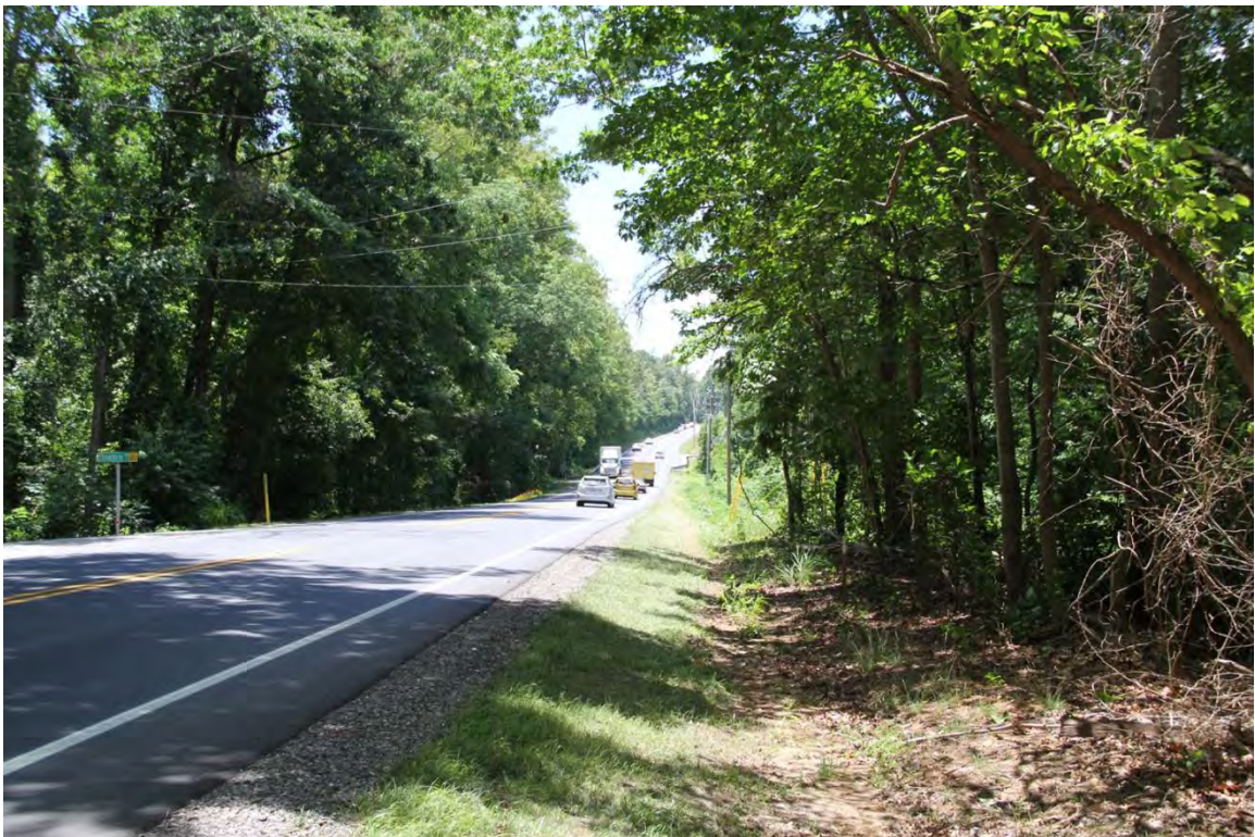
Sweeten Creek Road, south of Blue Ridge Parkway (#10), view to south
