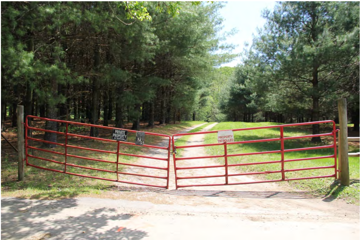
Entrance drive and gate, Round Top Road, view to south
