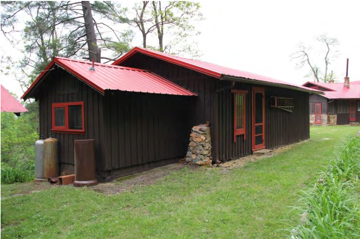
Garage, oblique rear view to northwest
