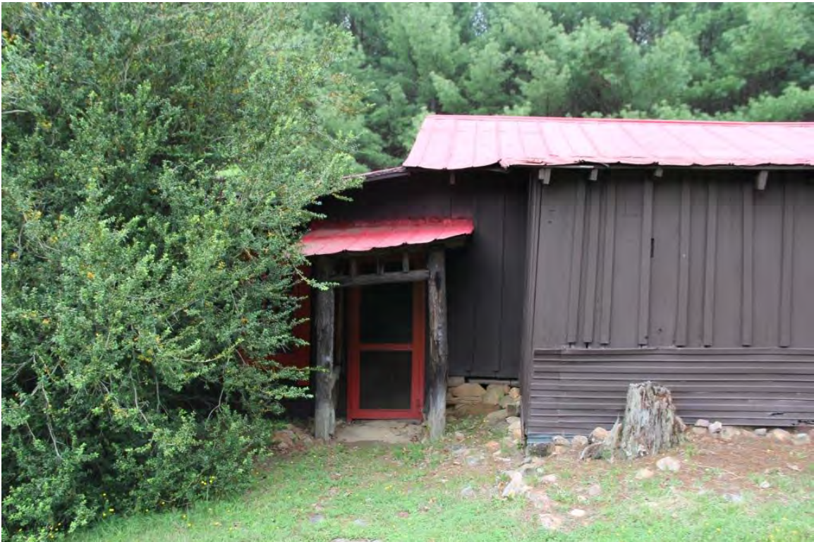
Garage, office entrance, view to north
