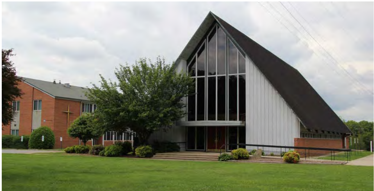
Arden First Baptist Church, 3839 Sweeten Creek Road, view to southwest
