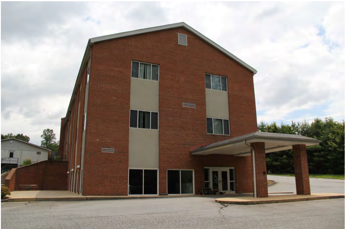
Youth building, rear elevation, view to east
