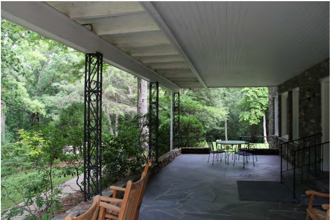
Givens House, front porch, view to northwest
