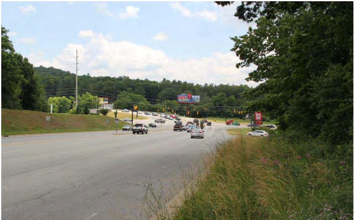
Airport Road (NC 280) near project beginning, view east to intersection with Hendersonville Road (US 25) and Sweeten Creek Road (US 25A)
