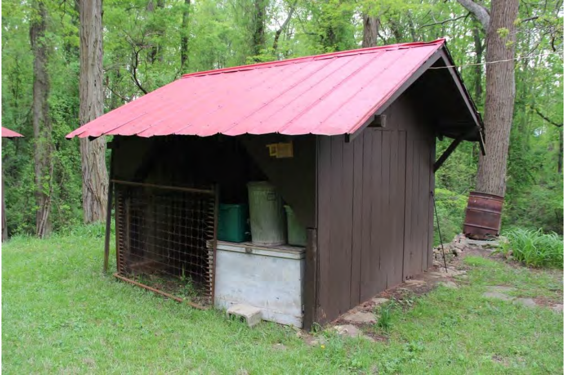
Shed, view to southwest
