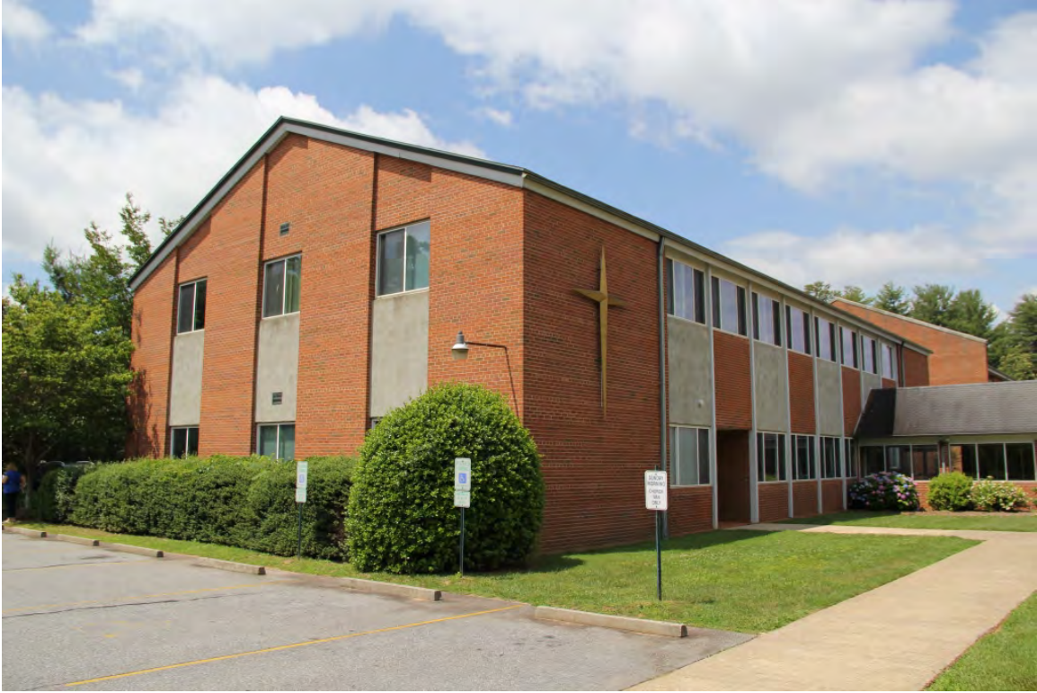
Education Building (original church structure), oblique front view to southwest
