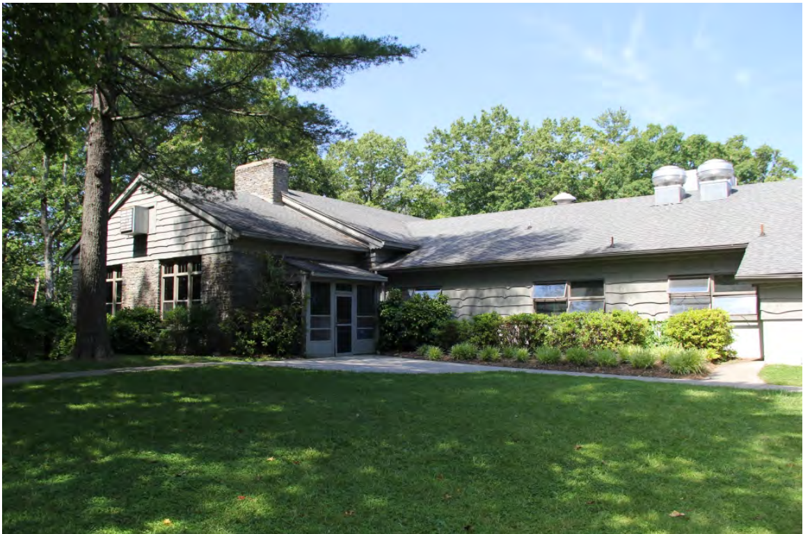
(#2) Lineberger Dining Hall (1951, enlarged 1958), view to southwest
