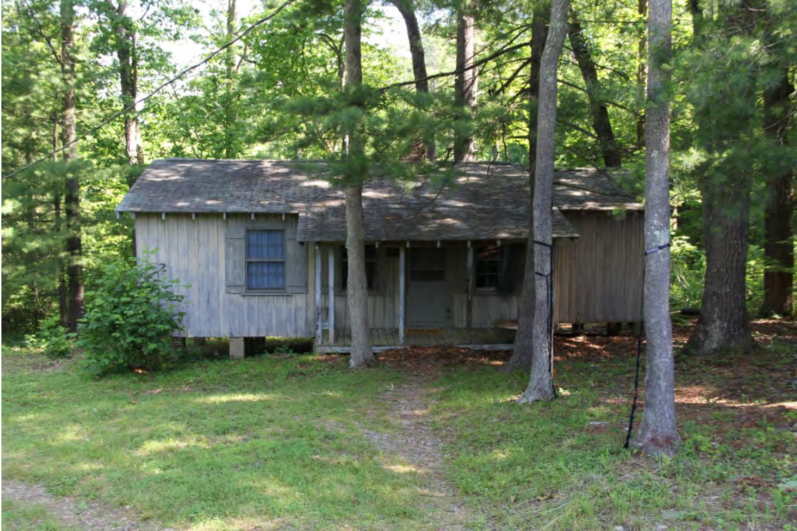
(#3) Cabin No. 2 (1951), façade, view to north
