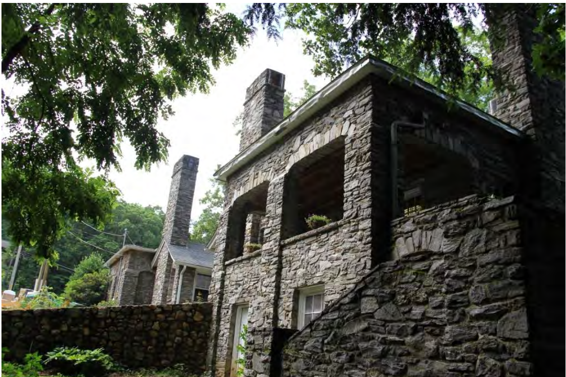
Givens House, oblique rear view to south
