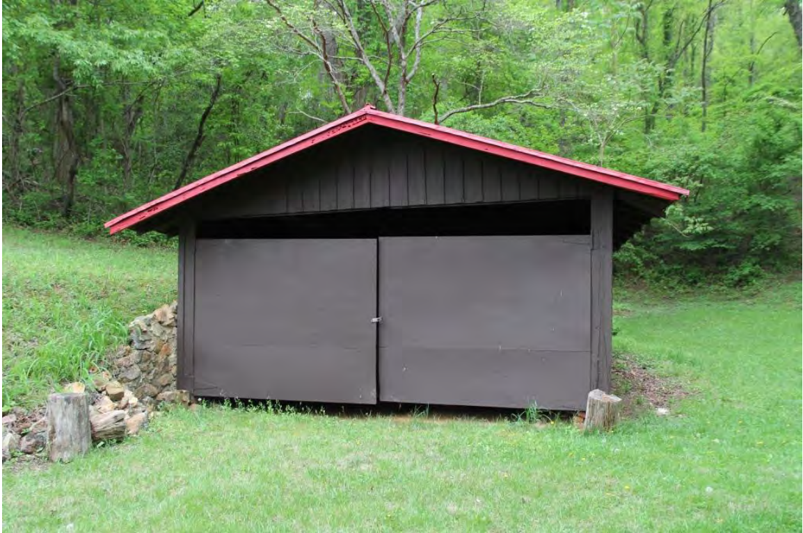
Barn, front elevation, view to east
