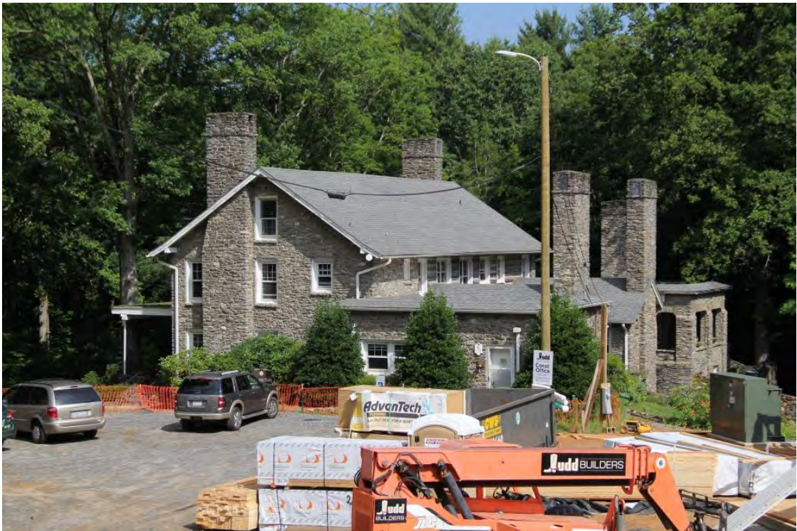
Givens House, oblique rear view to northwest
