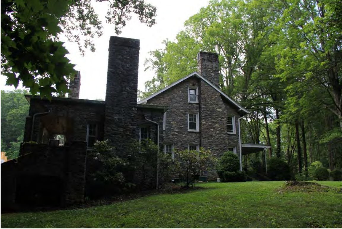
Givens House, northwest elevation, view to southeast
