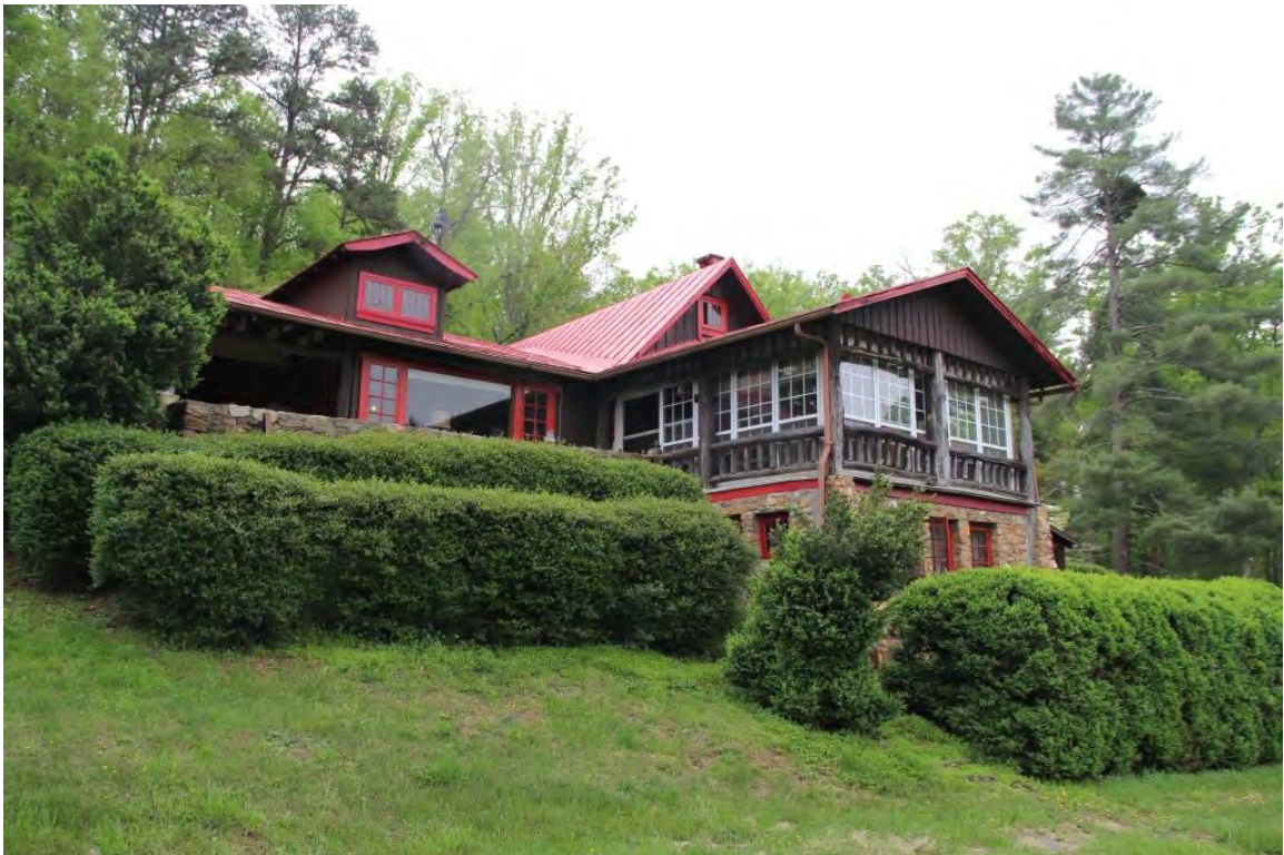
Horace W. and Emma Phillips House, oblique view to south
