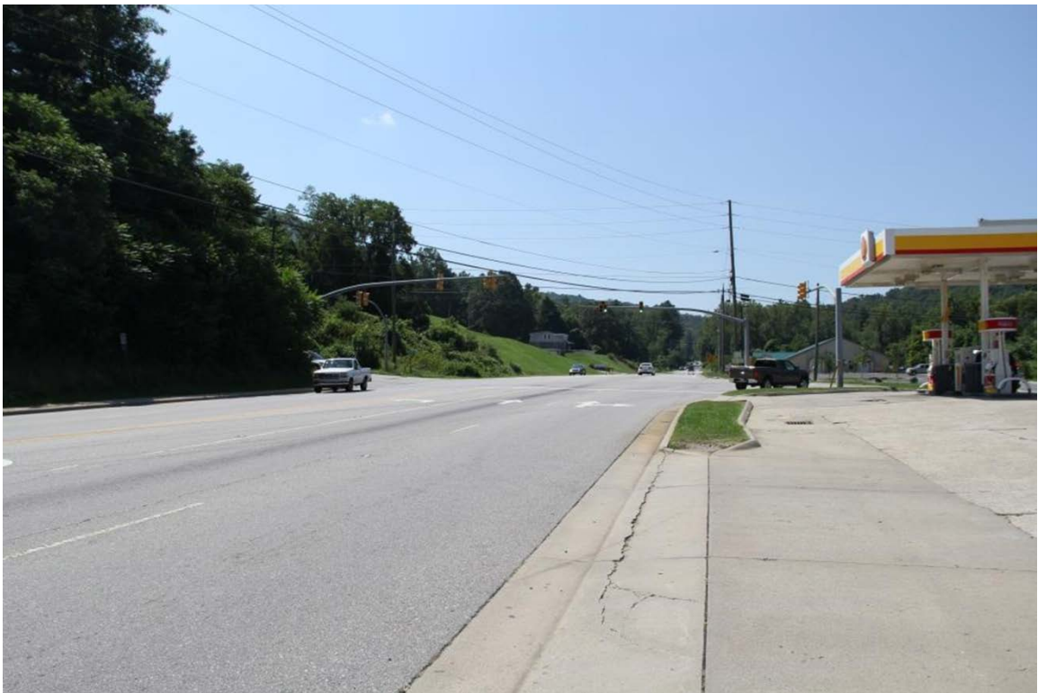
Project end, Sweeten Creek Road, view south to intersection with Rock Hill Road
