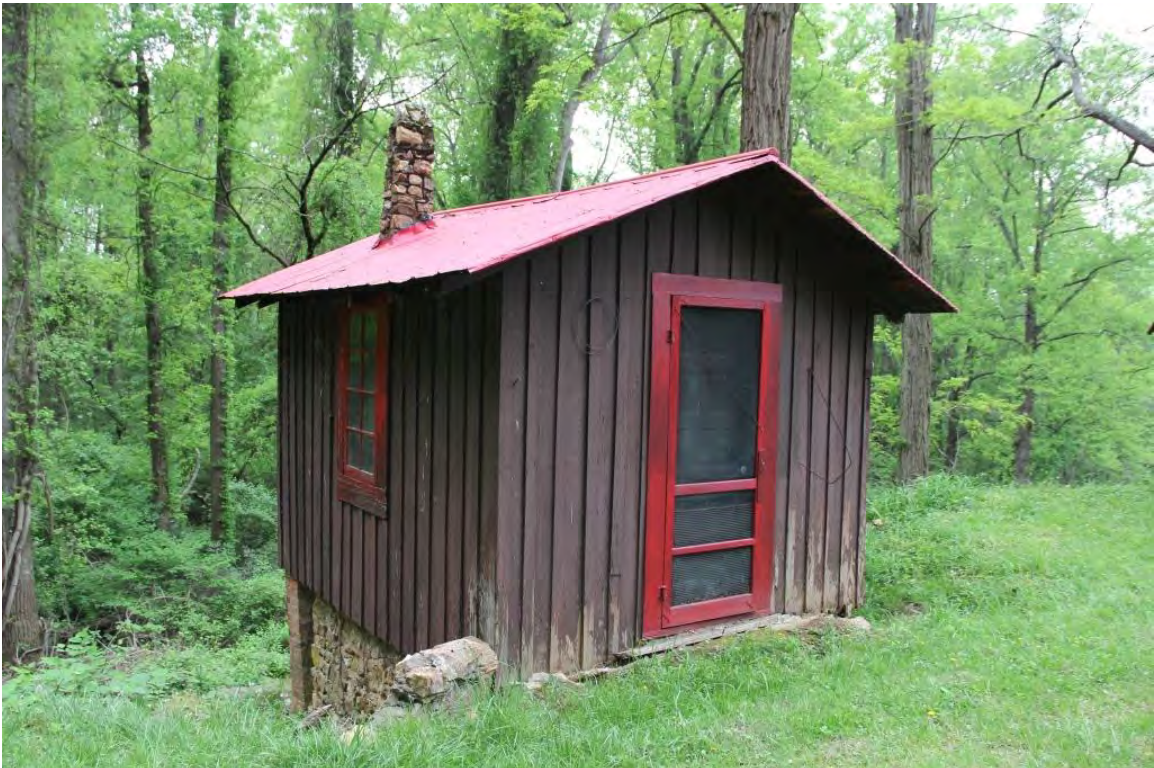
Servants' quarters, view to southwest
