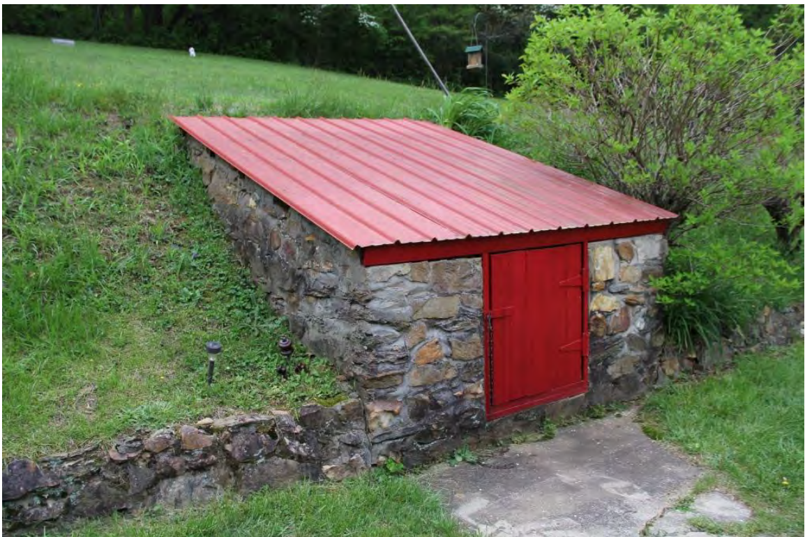
Coal bin, view to southeast
