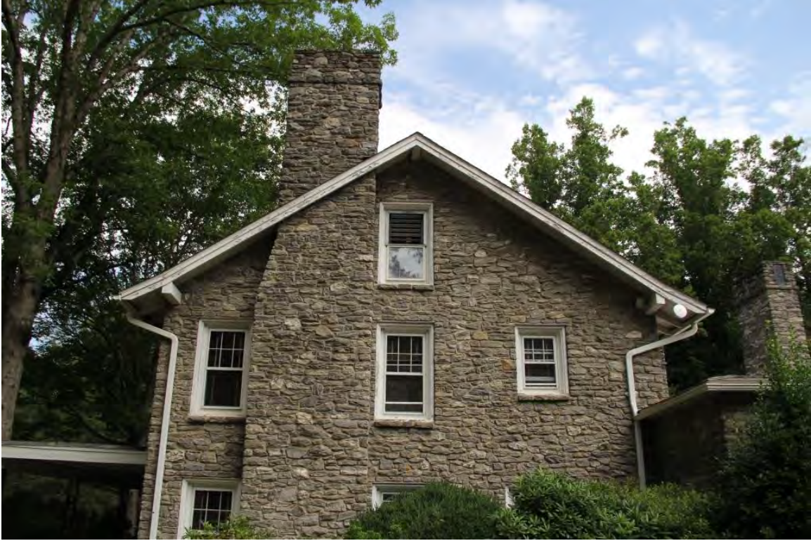
Givens House, southeast elevation, view to northwest
