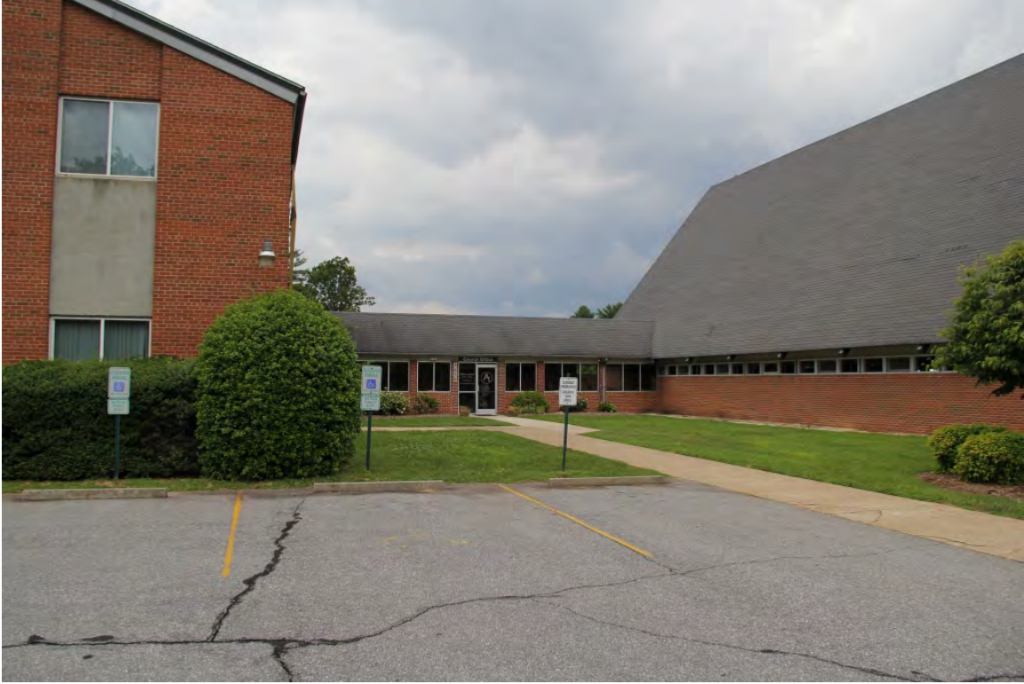
Entrance hall and office, facade, view to west
