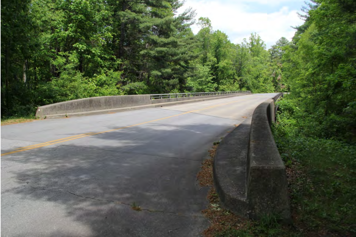
Blue Ridge Parkway, bridge over Sweeten Creek Road, view to northeast
