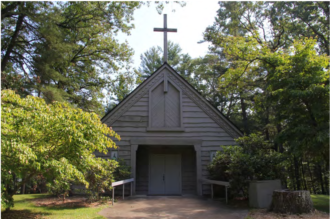
(#5) Whisnant Chapel (1953), façade, view to northeast
