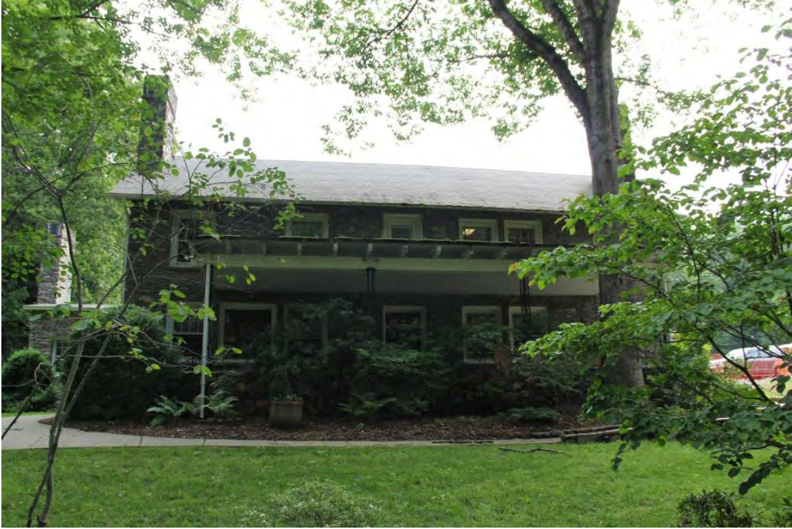
Givens House, façade, view to northeast
