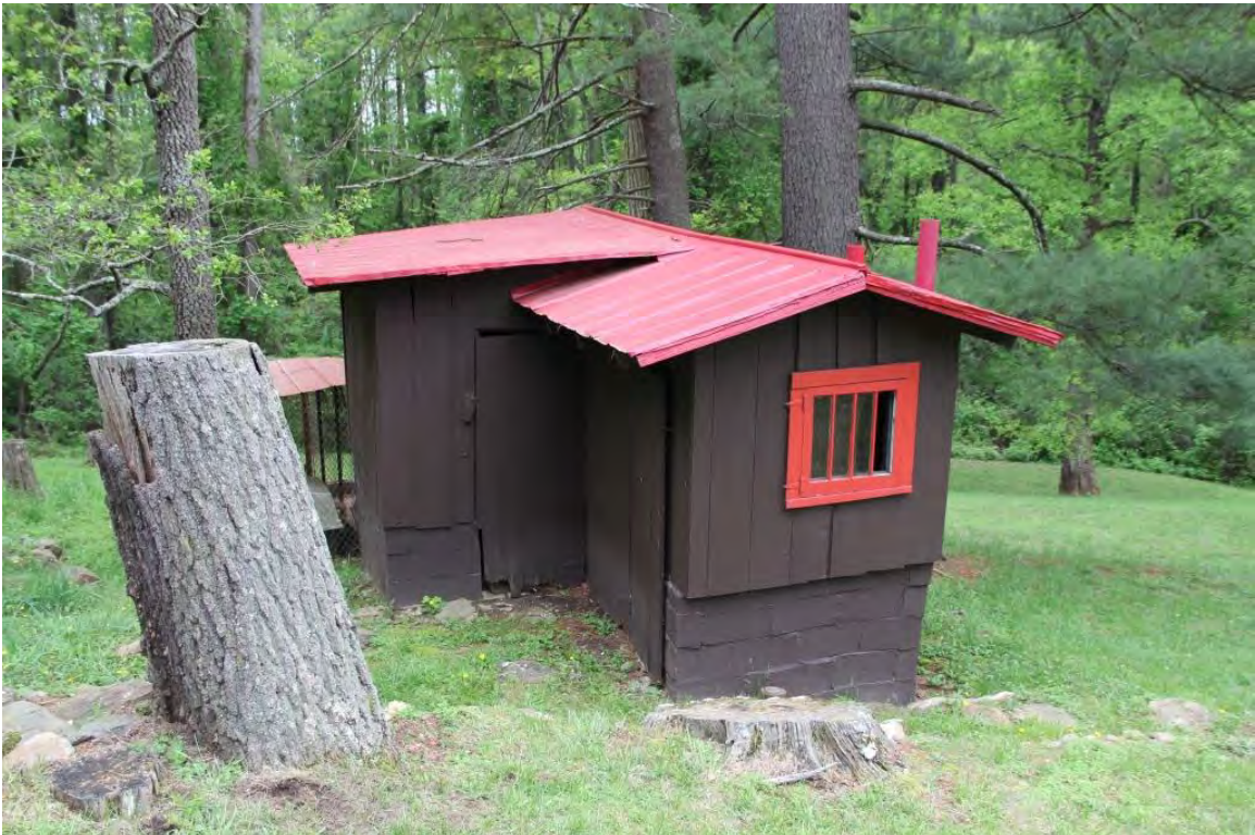
Servants' bath house, view to southwest
