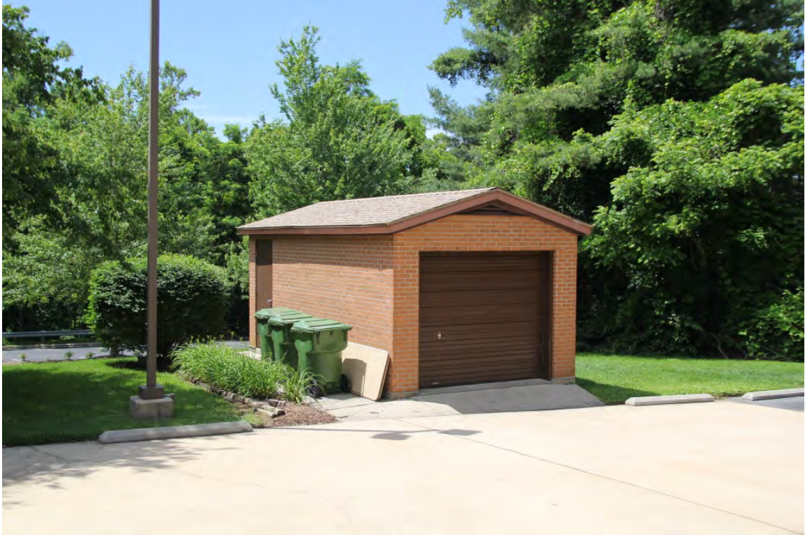
Garage, view to south
