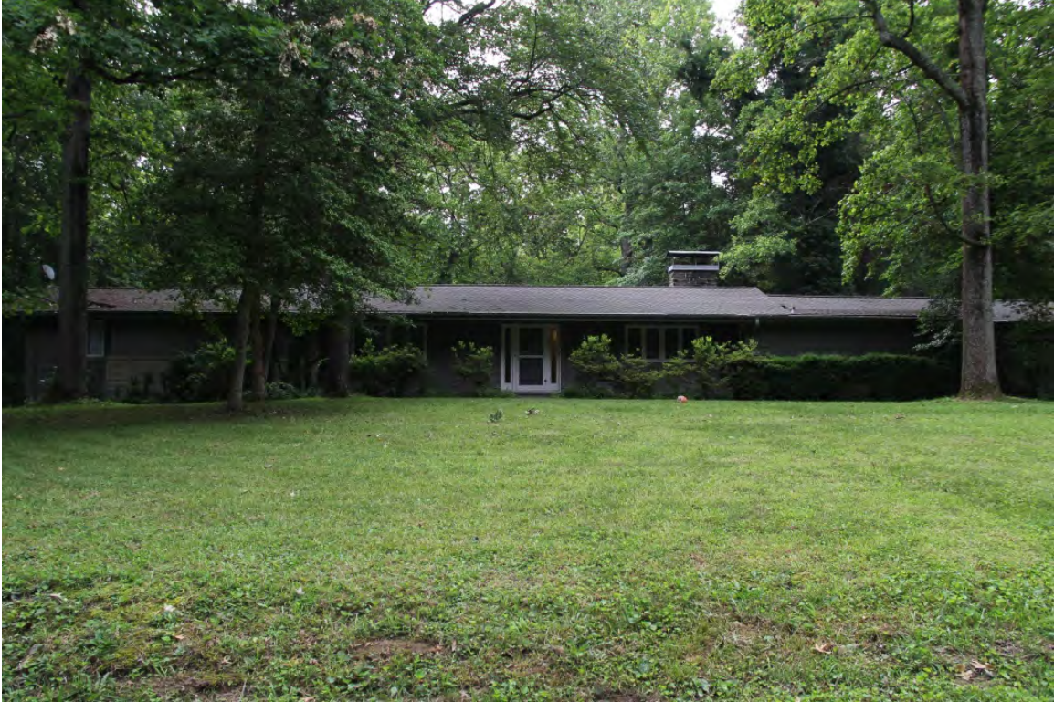
(#9) Director's Residence (1959), façade, view to southeast
