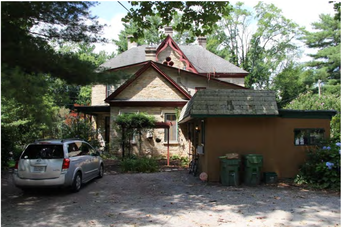
Blake House, rear elevation, view to southwest
