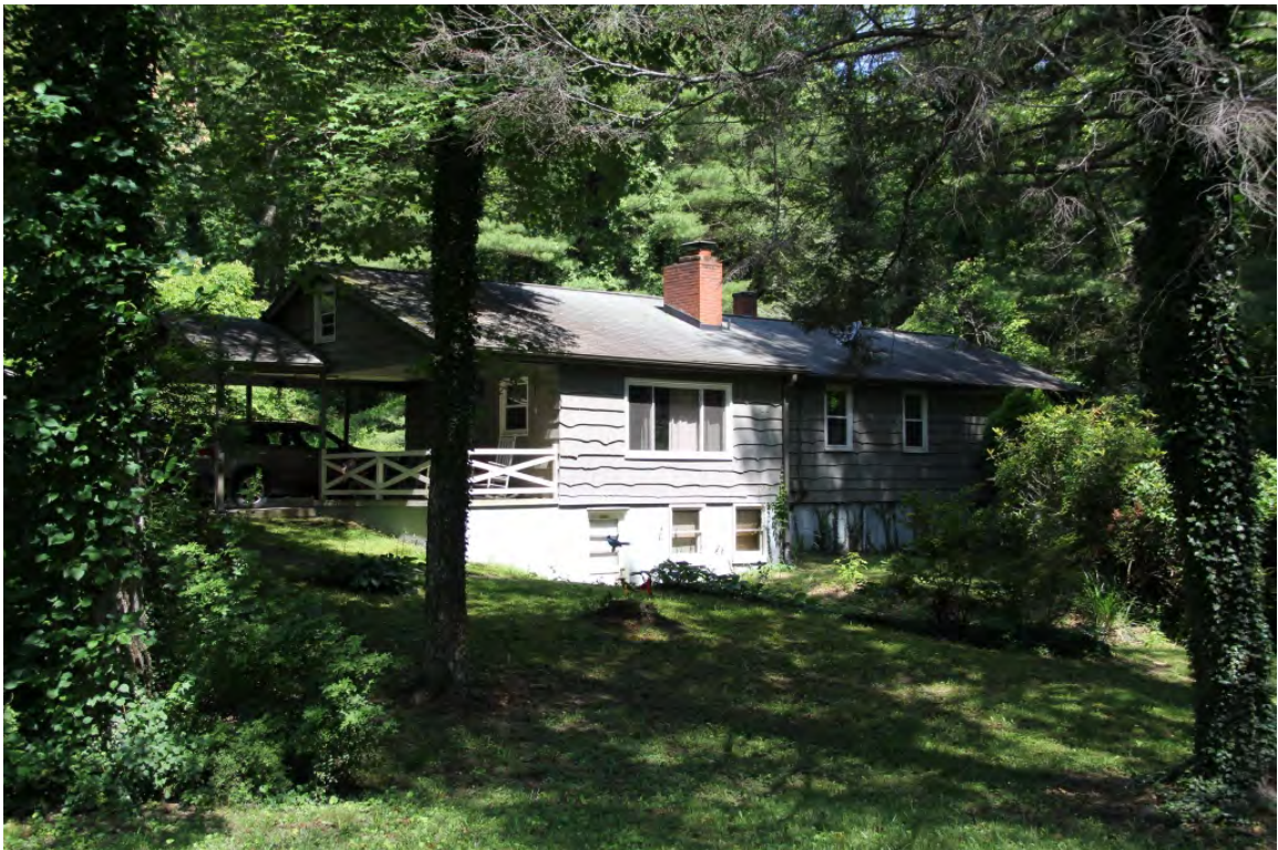
(#10) Caretaker's Residence (1952), oblique view to northwest
