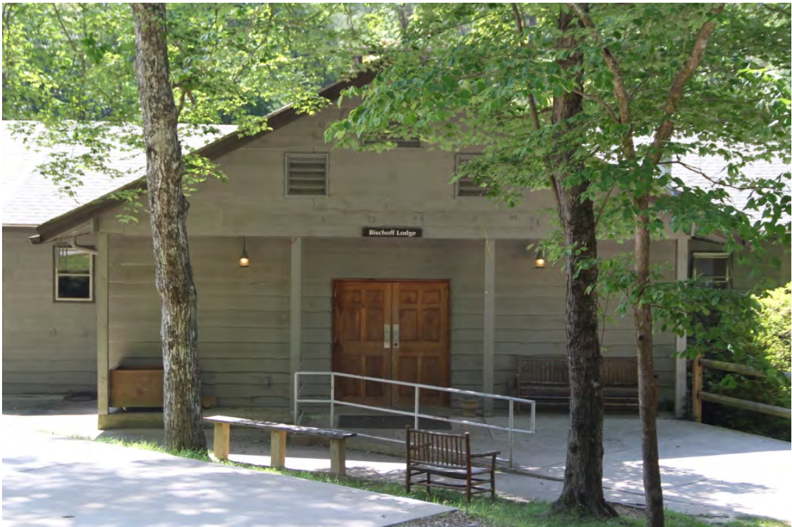
(#12) Bischoff Center (1966), façade, view to southeast
