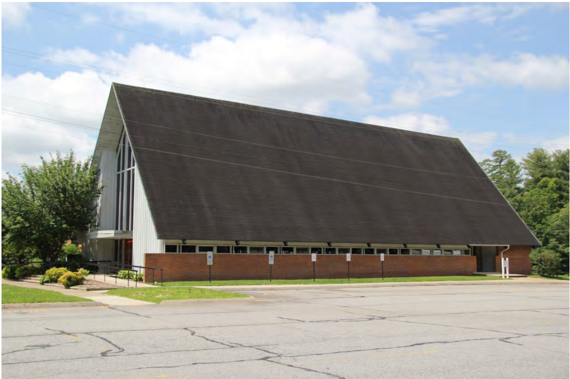
Sanctuary, oblique view to southwest
