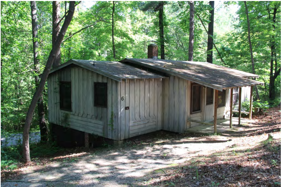
(#3) Cabin No. 6 (1951), view to east
