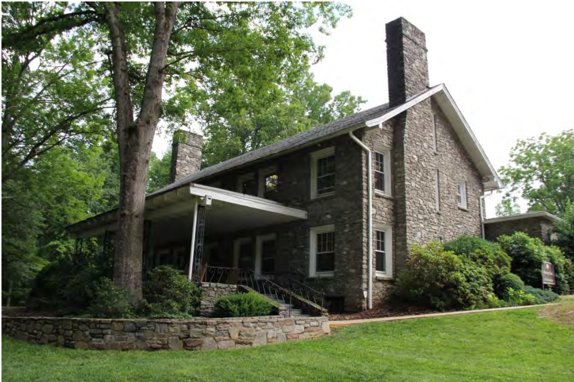
Dr. Maurice and Marion Givens House, 2360 Sweeten Creek Road, oblique front view to northwest
